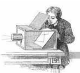
image 2. Principle of specular reflection (integrated in some types of professional cameras even today)
