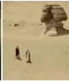
Image 21. Two Arabs near the unexcavated Sphinx - 1860
